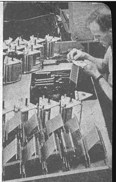
21 - ASSEMBLING OSCILLATOR TUNING CONDENSES
