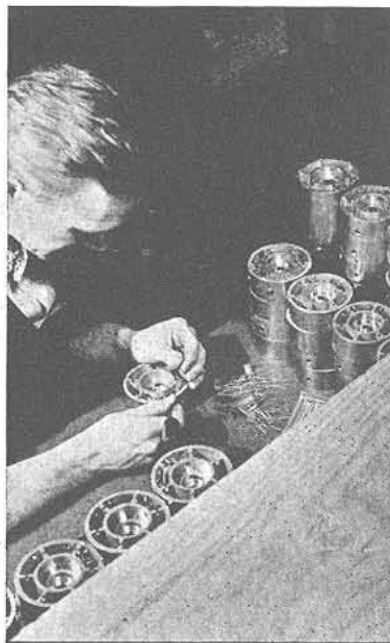
6 - ASSEMBLING ATTENUATOR HOUSINGS
