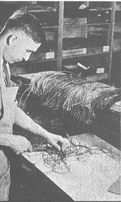
4 - FORMING MAIN WIRING CABLE
